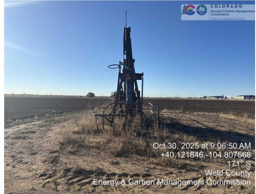
Photo 2 well head and equipment
