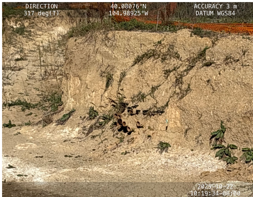
Open, exposed flowlines
