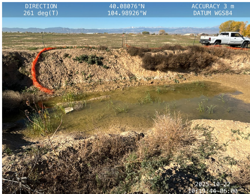
Groundwater within excavation
