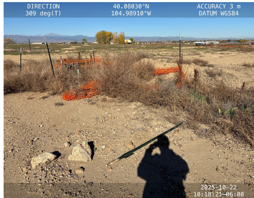
Weeds. Torn excavation fencing
