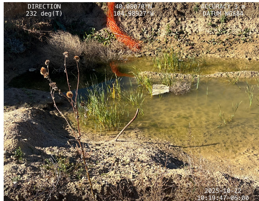
Groundwater within excavation
