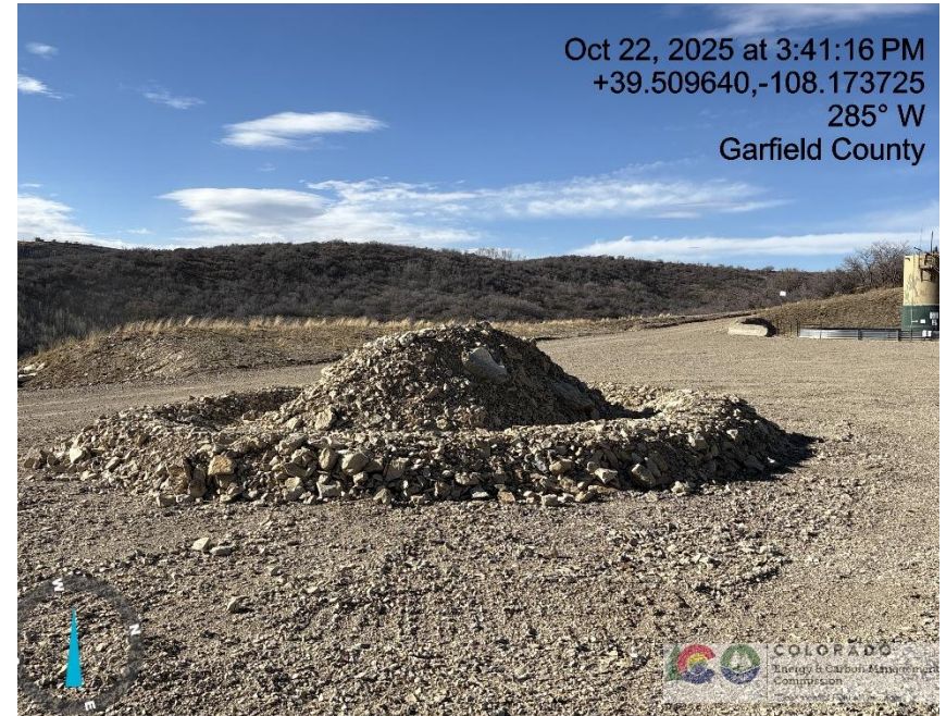
Photo # 1785 Soil & rock stockpile with berm
