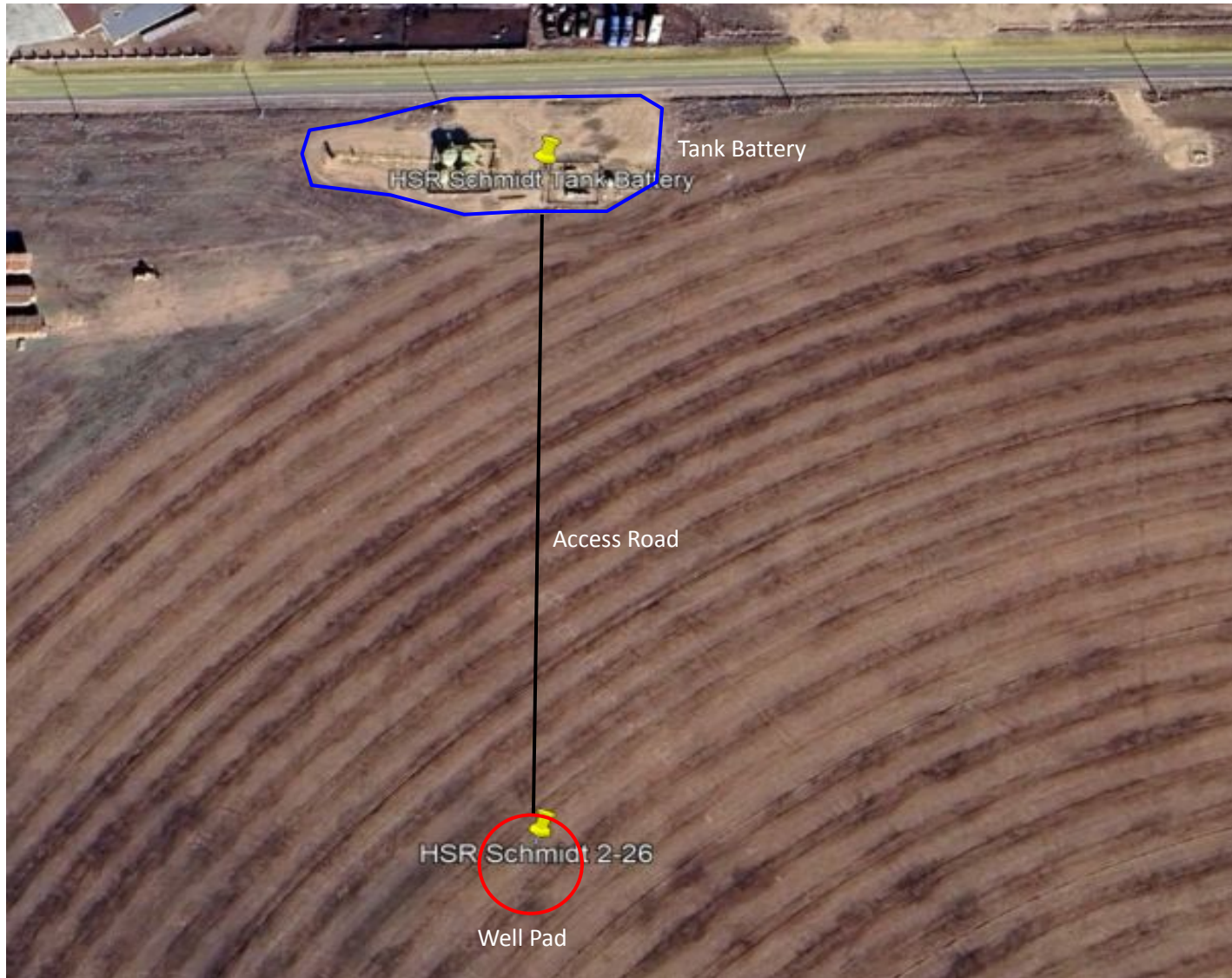
Photo 1. 2025 aerial imagery showing the Tank Battery location (highlighted in blue), Access Road (highlighted in black) and well pad (highlighted in red).
