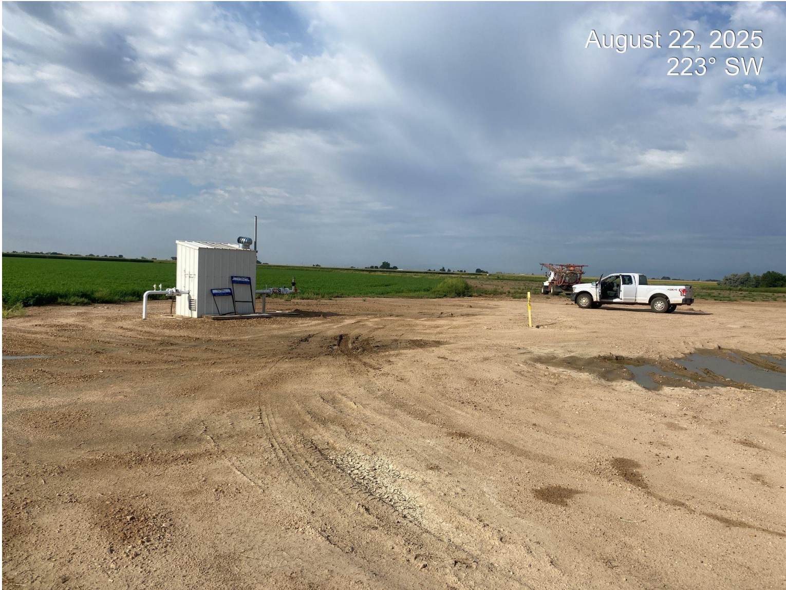
Photo 3. View of tank battery taken from the western edge facing east. Note: disturbance remains with gravel, meter shed has not been removed, Well location signs also remain on location.
