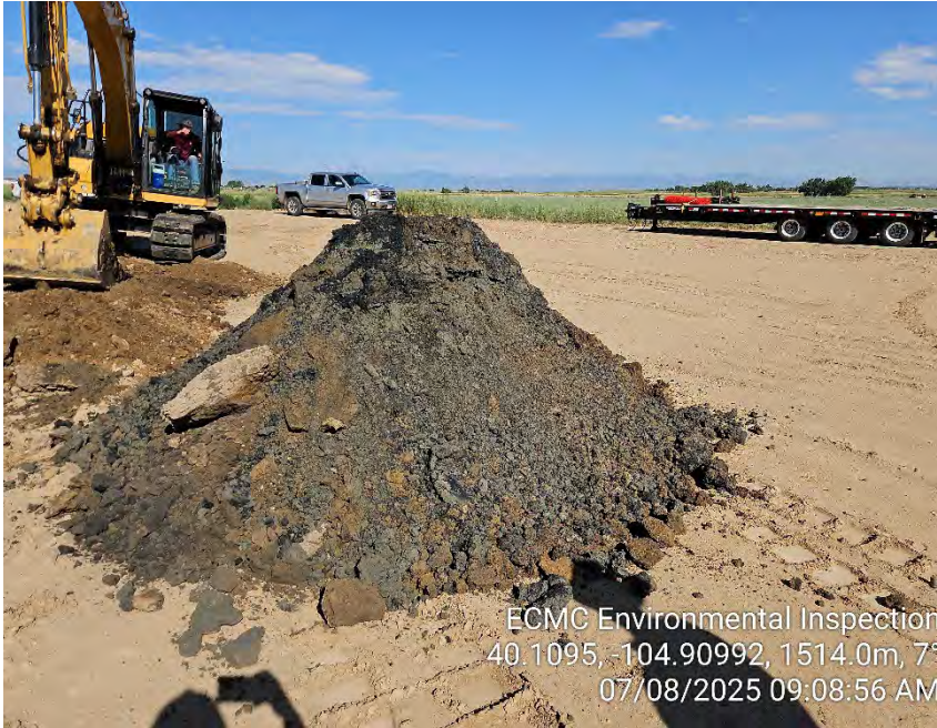
Photo 7 – Impacted soil excavated from pothole adjacent to pipelines/flowlines. Fence down for active work
