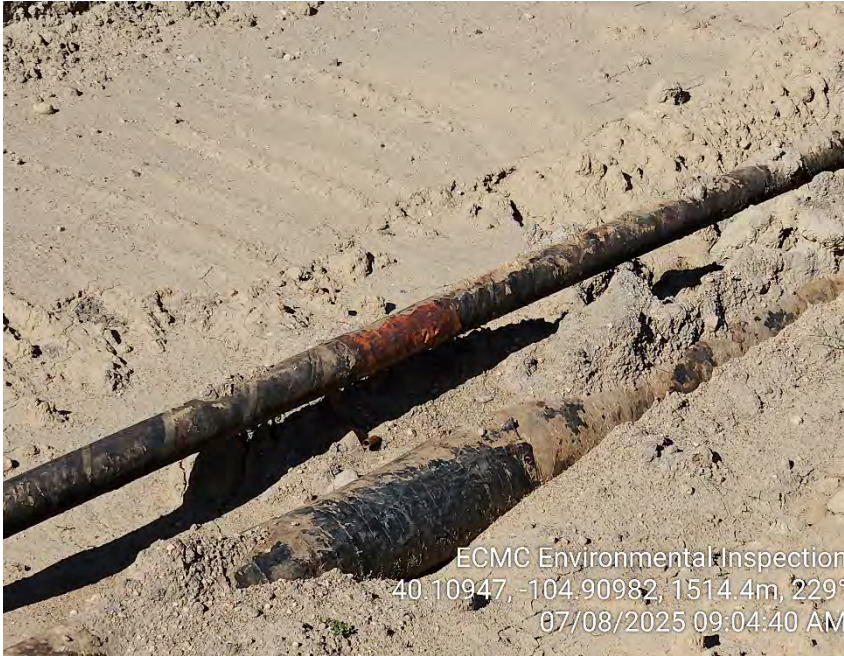
Photo 3 – Pipelines/flowlines in open excavation
