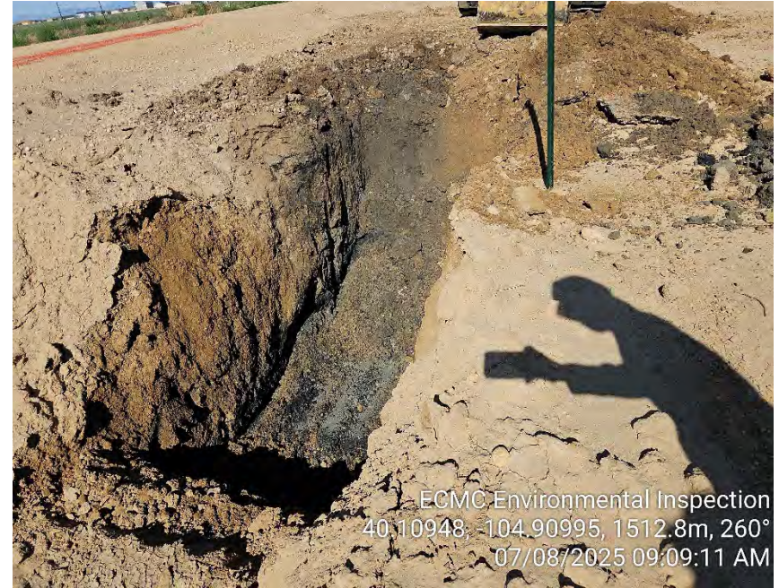
Photo 6 - Pothole adjacent to flowline shows impacted soil. Fence down for active work.
