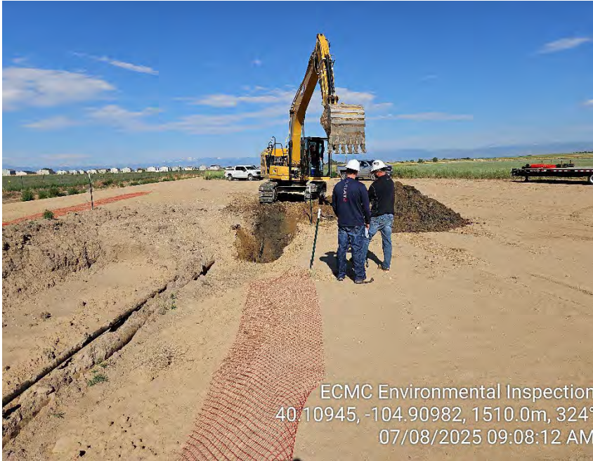
Photo 5 – Pothole adjacent to flowline shows impacted soil. Fence down for active work.
