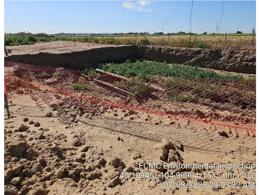
Photo 2 - Spill excavation with pipelines/flowlines
