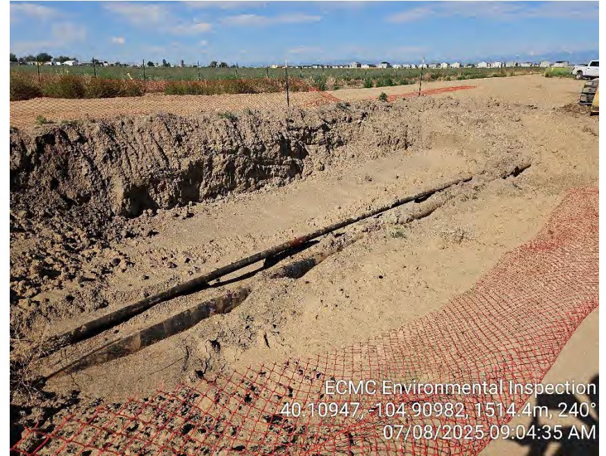
Photo 4 - Spill excavation with pipelines/flowlines. Fence down for active work
