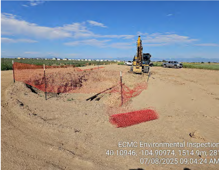
Photo 1 – Spill excavation with pipelines/flowlines. Fence down for active work
