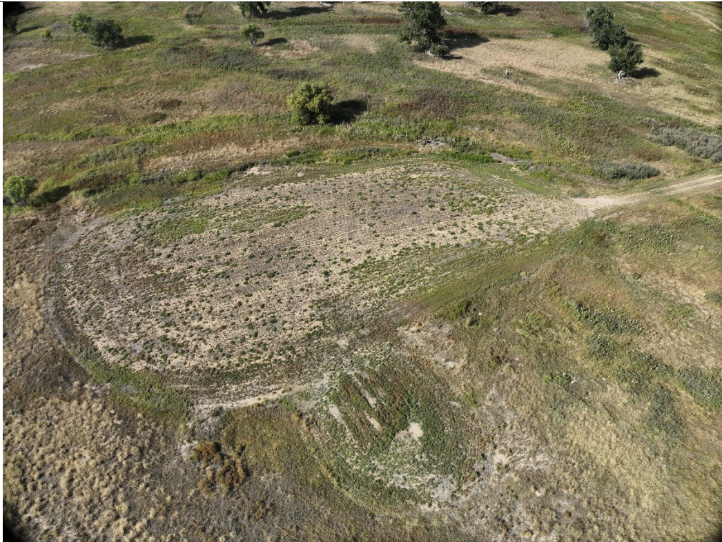
In View – Pad, Access Road (Variance Requested)
