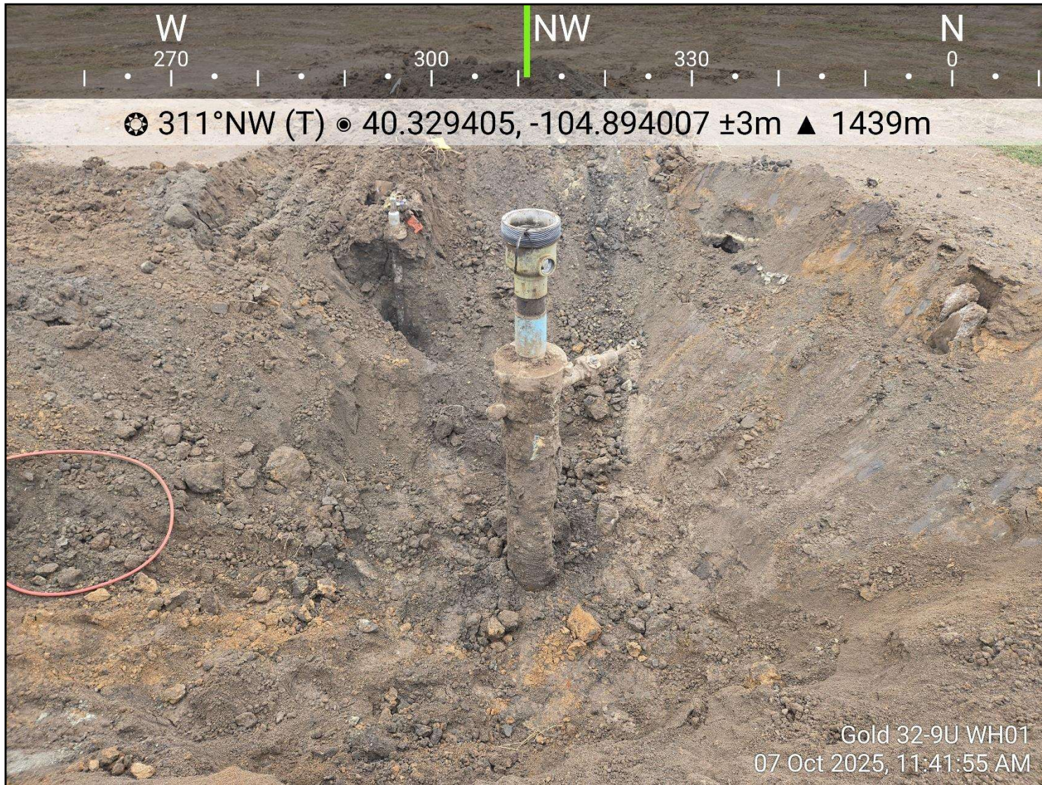
Photo 5: View of excavation extent, facing northwest
