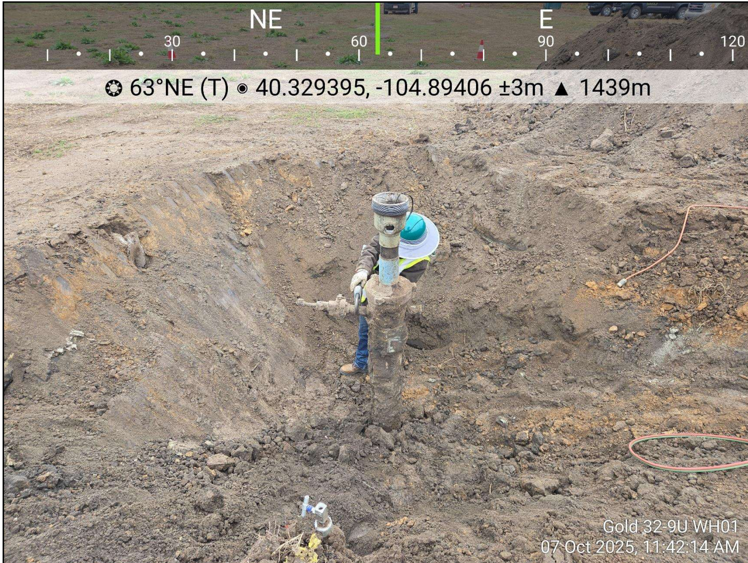
Photo 3: View of excavation extent, facing east-northeast
