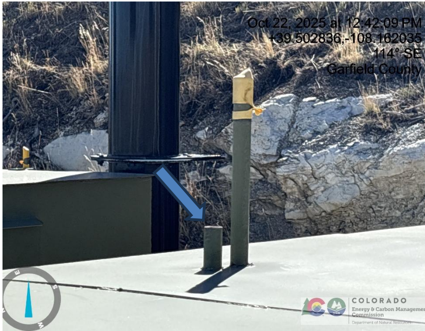
Photo # 1207 Rupture disc vent line does not comply with CECMC pressure safety device rules
