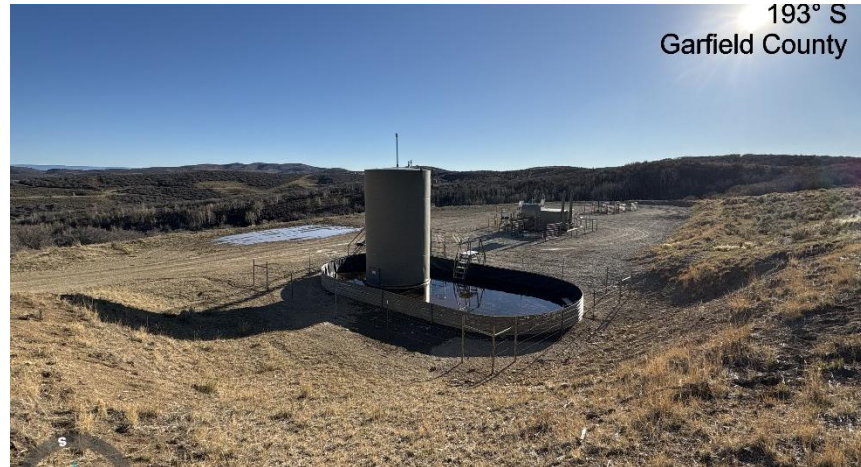
North East corner of location.
