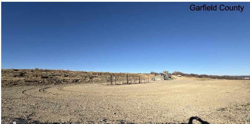
South West corner of location.
