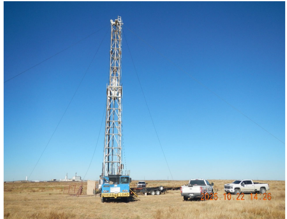
2. View of well location with Work-Over Rig rigged up over wellbore.
