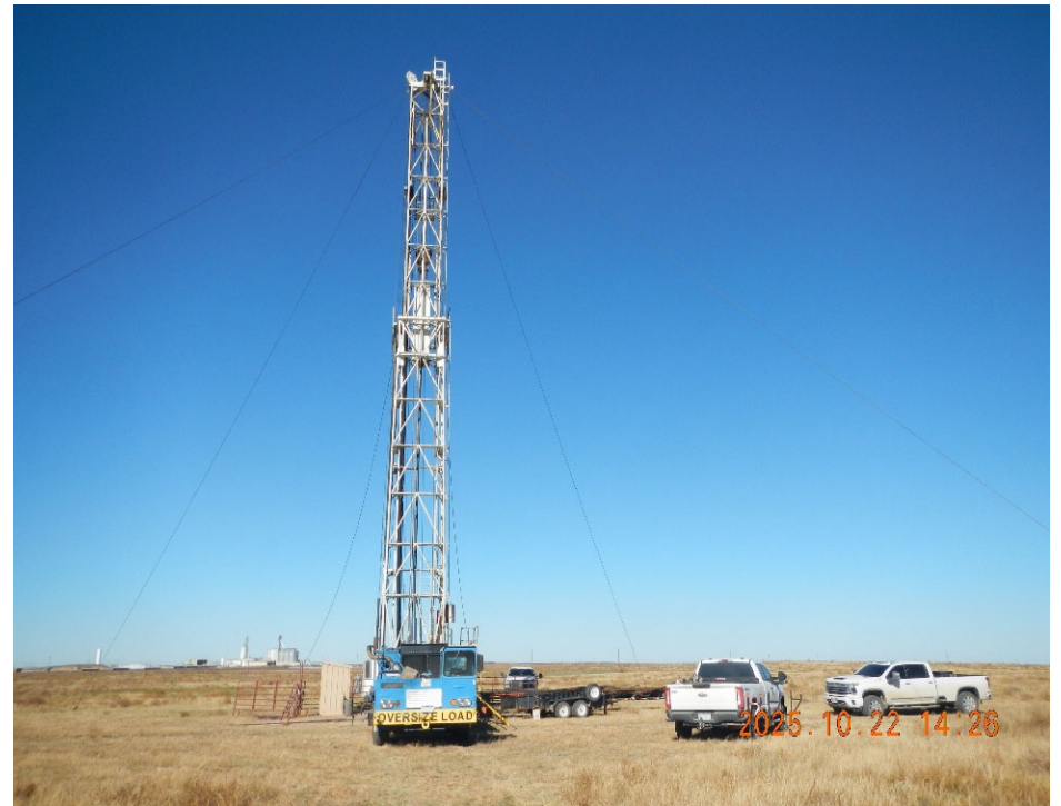
4. Well location overview. Work-over Rig rigged up over wellbore.
