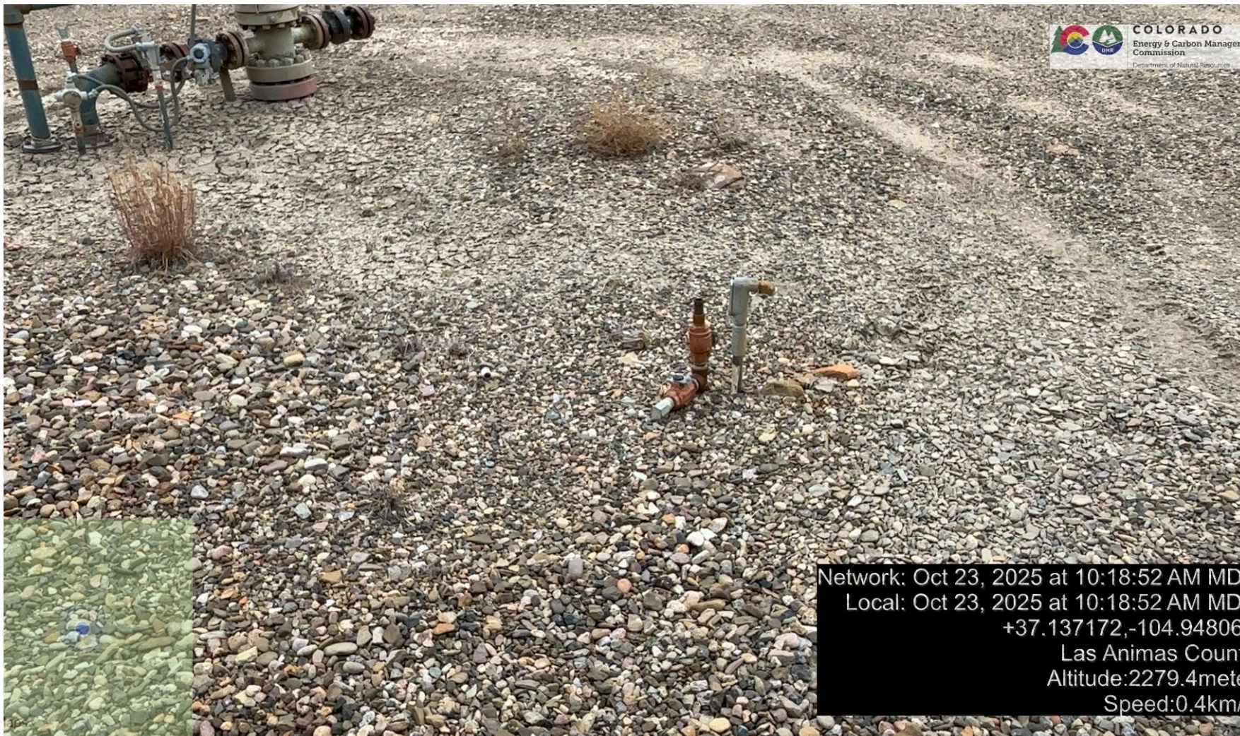
PHOTO 3: UNUSED EQUIPMENT (1" RISER). REMOVE OR MARK RISER PER RULE 606. CA DATE 11-23-2025.
