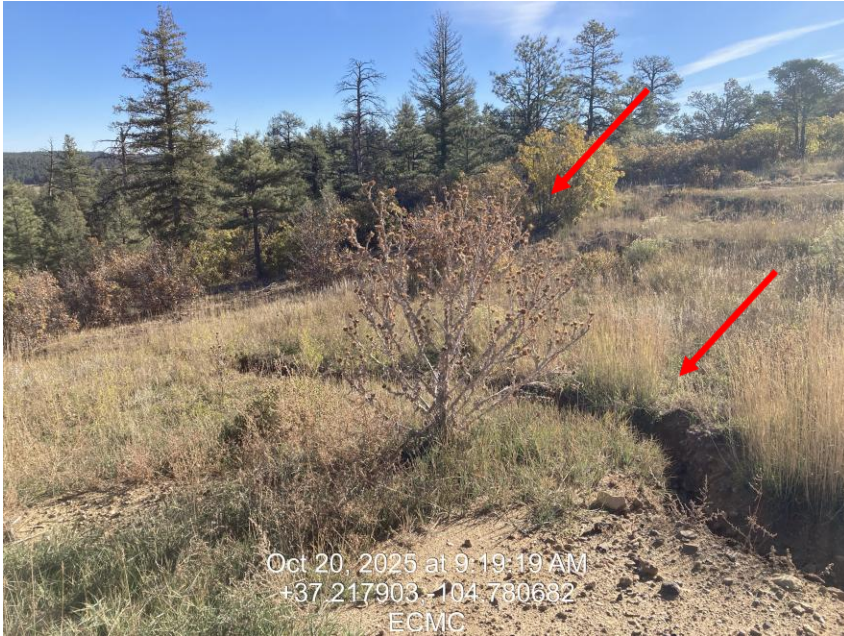
Photo 5 – Erosion and Noxious Weeds
