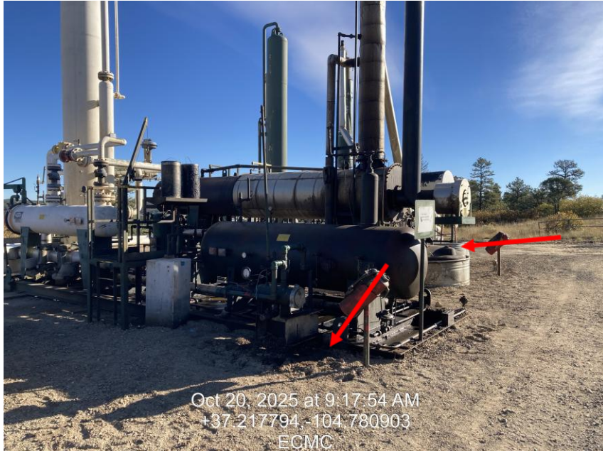
Photo 3 – Impacted soils at arrow and between Dehydration Units
