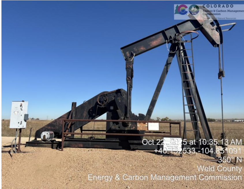
Photo 1 well head and equipment
