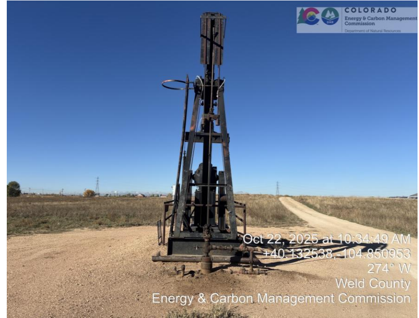
Photo 2 well head and equipment
