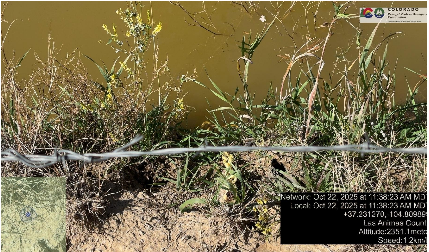
PHOTO 3: THERE IS LESS THAN 2' FREEBOARD. Lower fluid level so at least two feet of freeboard exists per Rule 909.c. CA DATE 10-23-2025.
