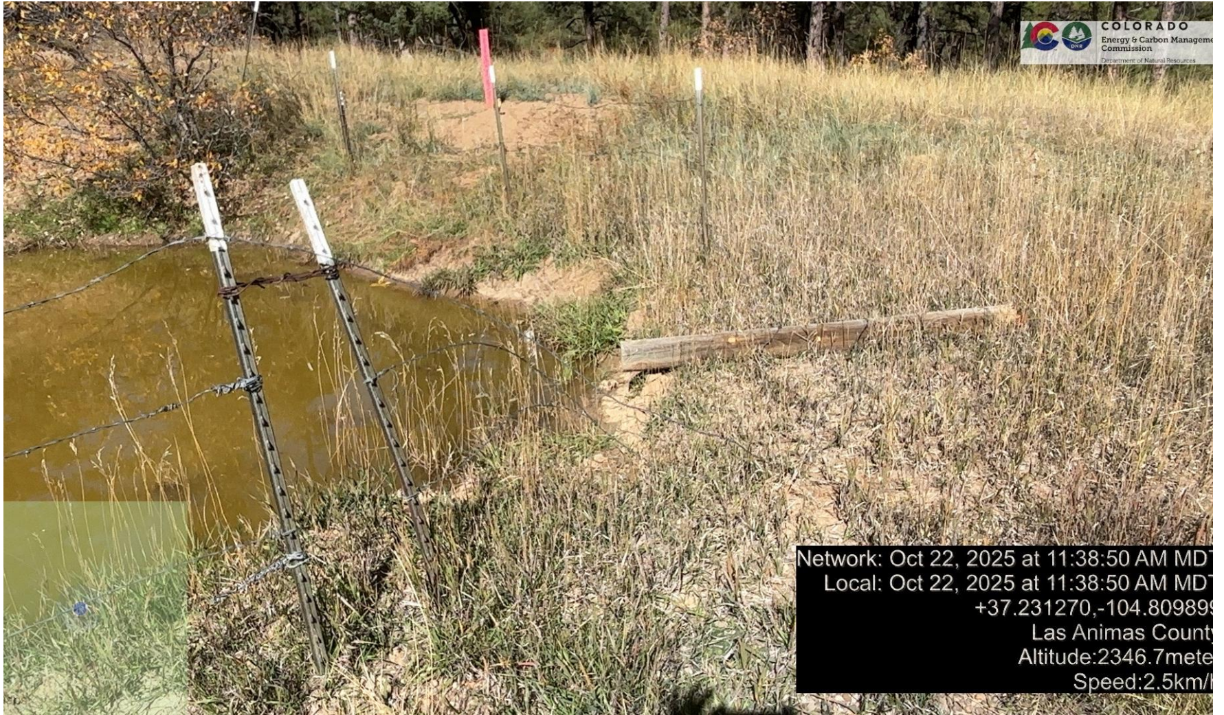
PHOTO 4: FENCE AROUND PIT IS IN DISREPAIR. REPAIR FENCE ALL THE WAY AROUND PIT PER RULE 1002. CA DATE 11-22-2025.
