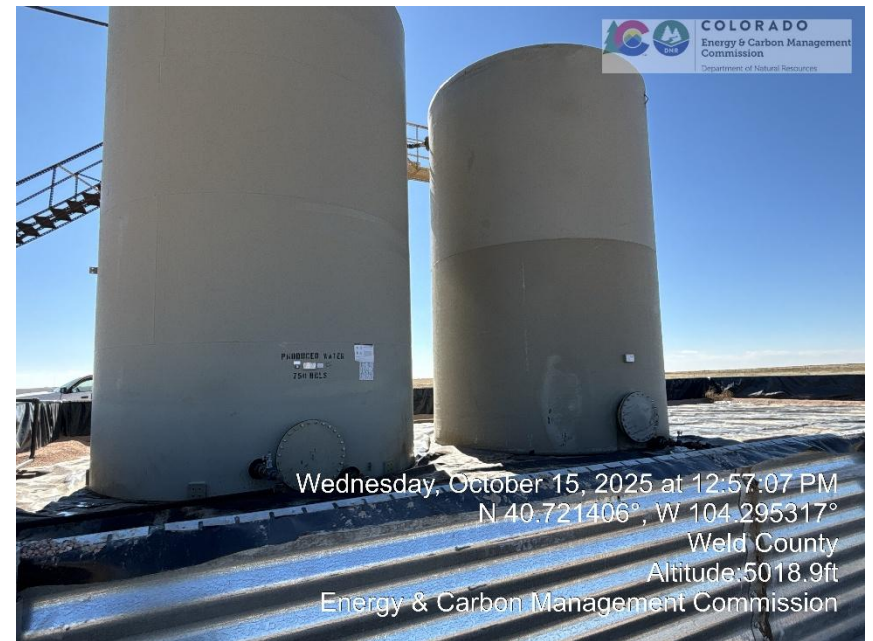
Photo 4 – Tank NFPA, Content and Capacity Labels are missing
