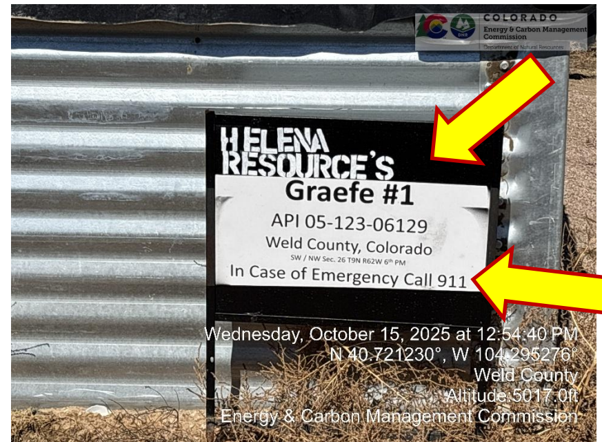
Photo 2 – Tank Battery Sign – missing 24 Hour Emergency Contact Number
