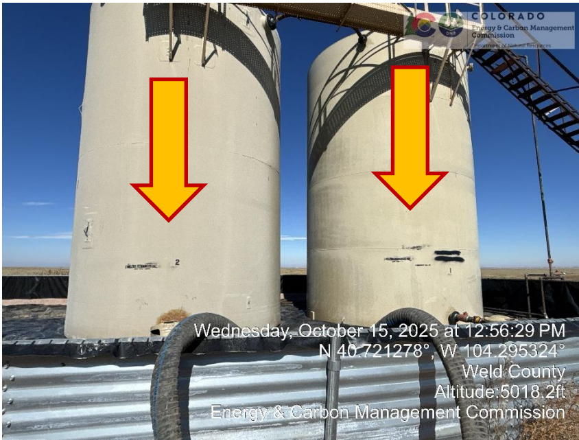
Photo 3 – Tank NFPA, Content and Capacity Labels are missing
