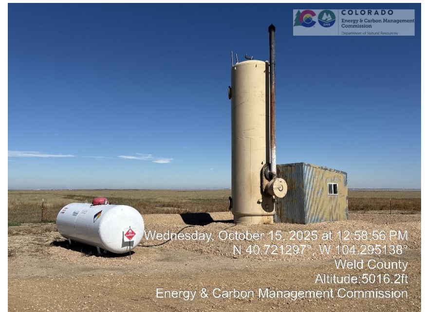
Photo 6 – Heater Treater and Propane Tank
