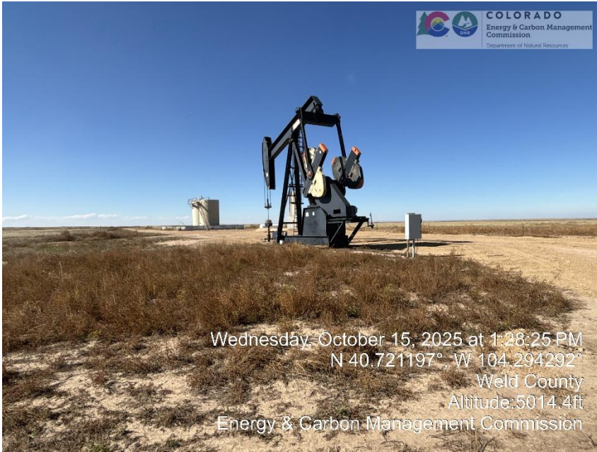
Photo 9 – Pumping Unit – Weeds/Debris
