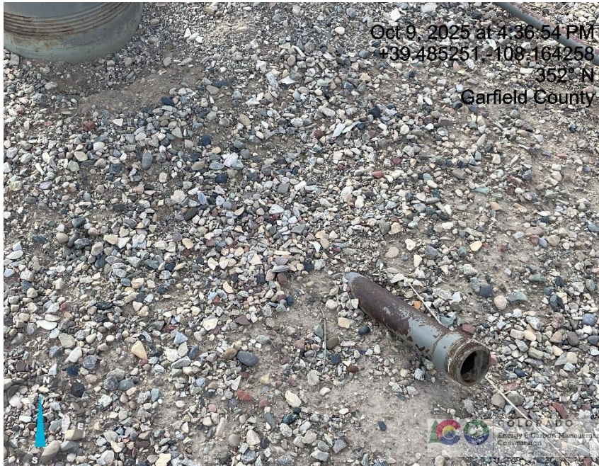
Photo # 5979 Open ended piping near wellhead/wildlife hazard/available for entry by wildlife
