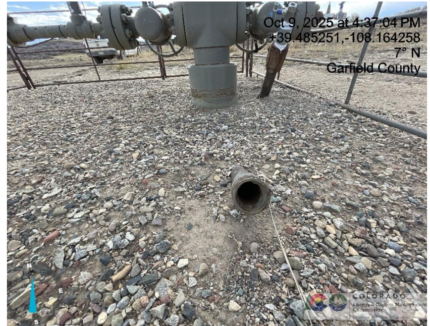
Photo # 5980 Open ended piping near wellhead/wildlife hazard/available for entry by wildlife
