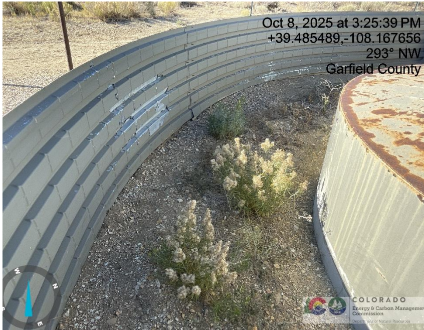
Photo # 5063 Weeds/undesirable plant species in secondary containment
