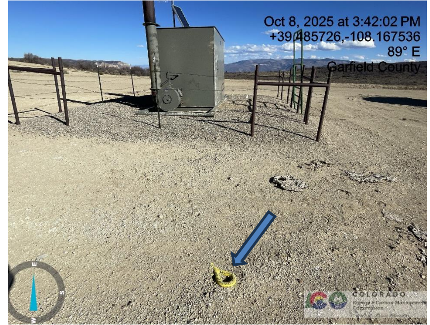
Photo # 5072 Same unmarked deadman
