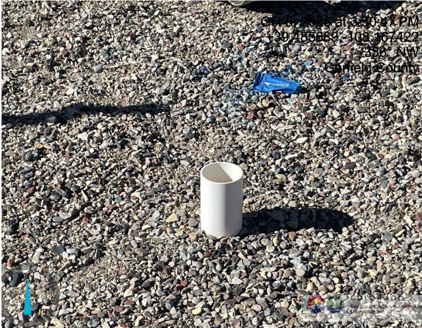
Photo # 5065 Open ended pipe near separator/wildlife hazard/available for entry by wildlife
