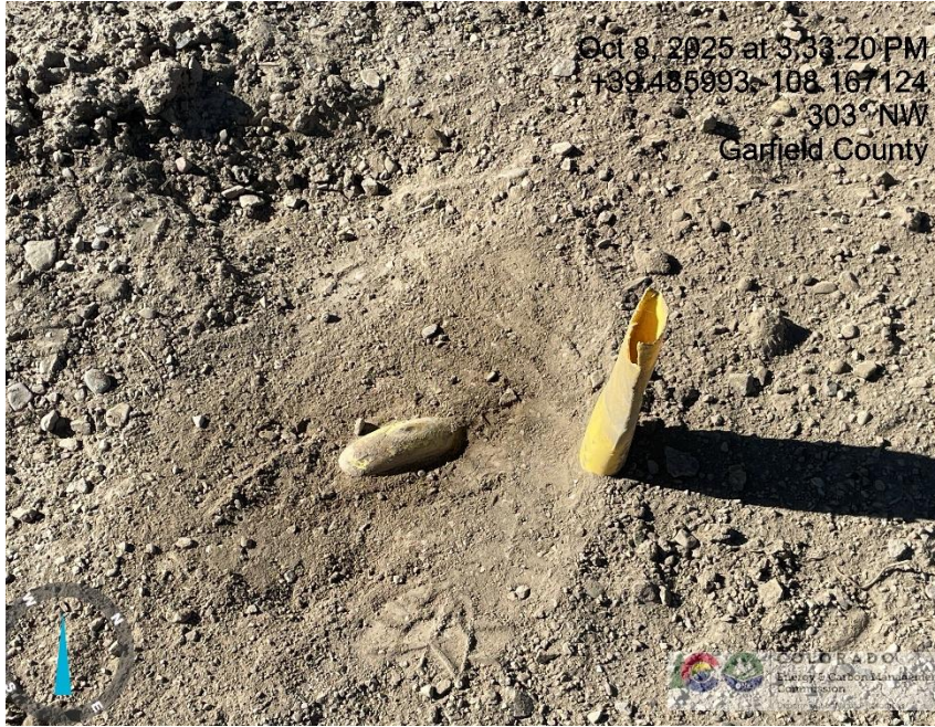
Photo # 5067 Improperly marked deadman
