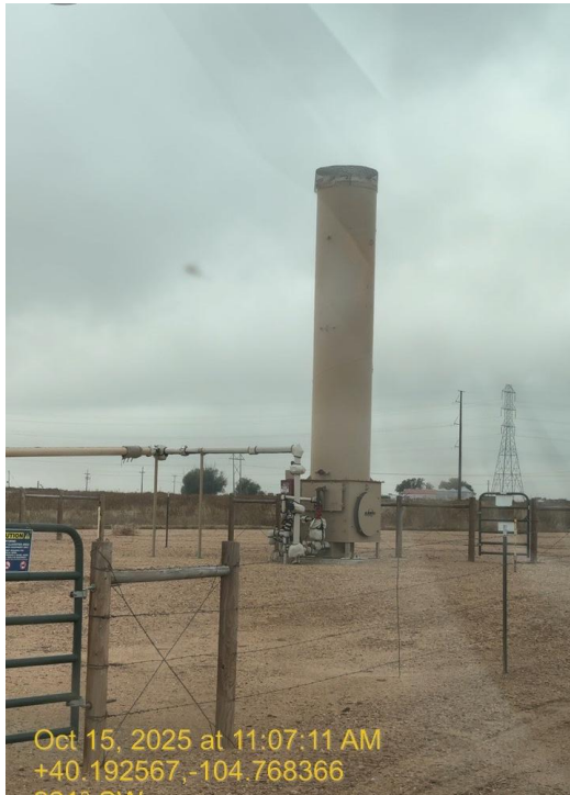
ECD on West Side of Location
