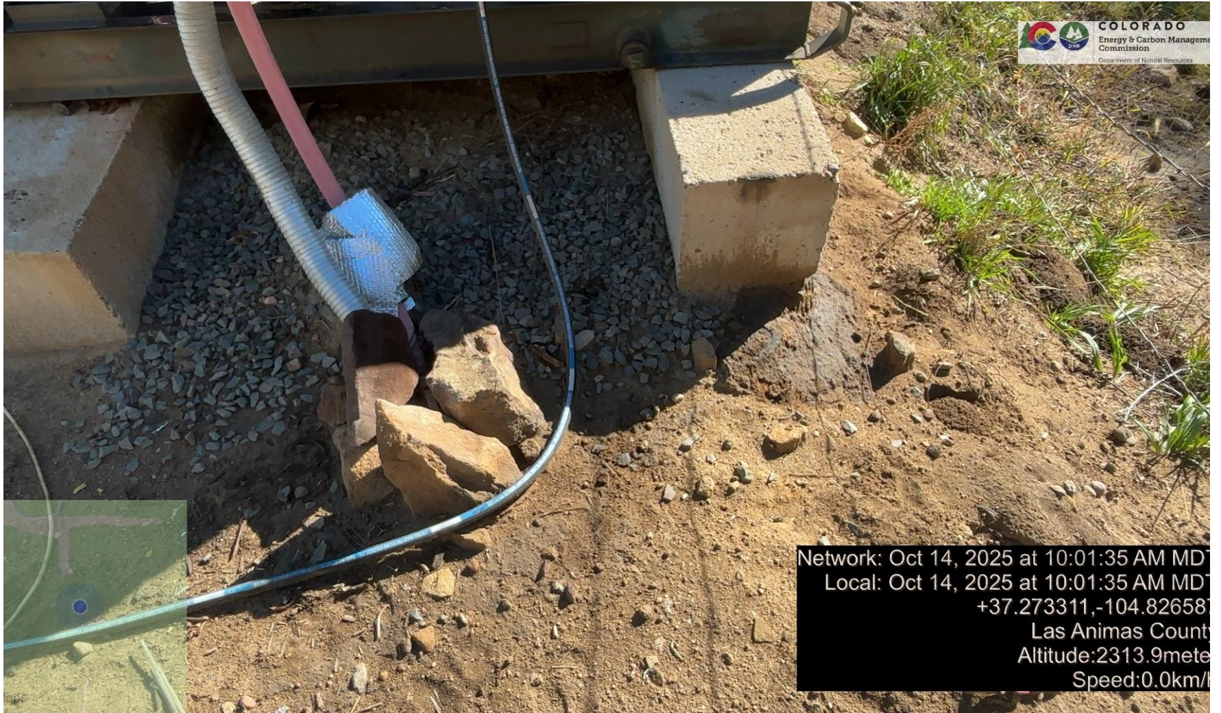
PHOTO 4: AREA OF IMPACTED SOIL NEAR PRIME MOVER. Conduct maintenance on equipment, cleanup stained material and review self inspection processes. COMPLY WITH RULE 1002,(2).D. CA DATE 11-14-2025.
