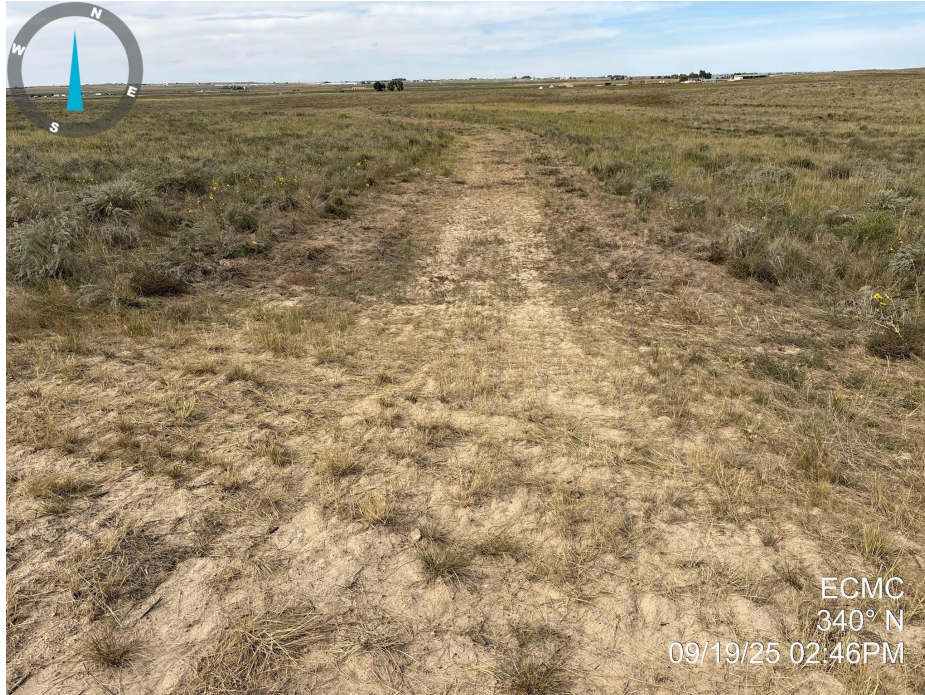
Photo 5. Photo taken of the access road to the well location, facing north, towards the location. Photo illustrates that final reclamation activities have taken place, with evidence of drill row seeding, but gravel remains and vegetation has not established to Rule 1004 standards.
