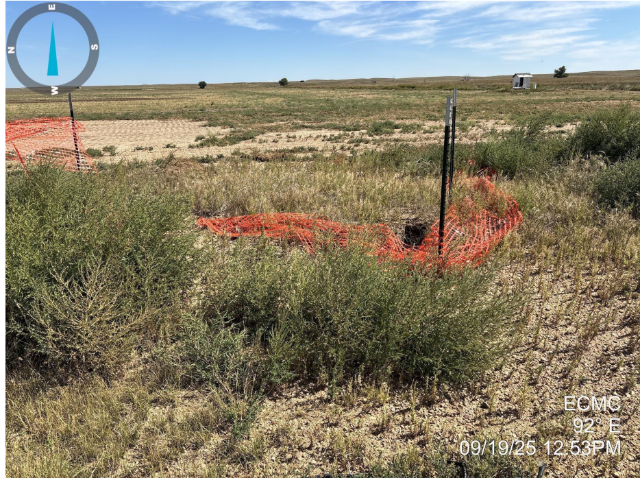
Photo 4. Photo taken of the tank battery location, facing east. Photo illustrates that fencing is in disrepair.
