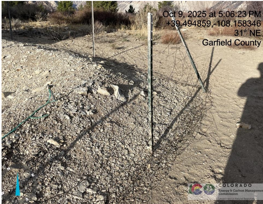
Photo # 6043 Fencing around tank battery needs maintenance
