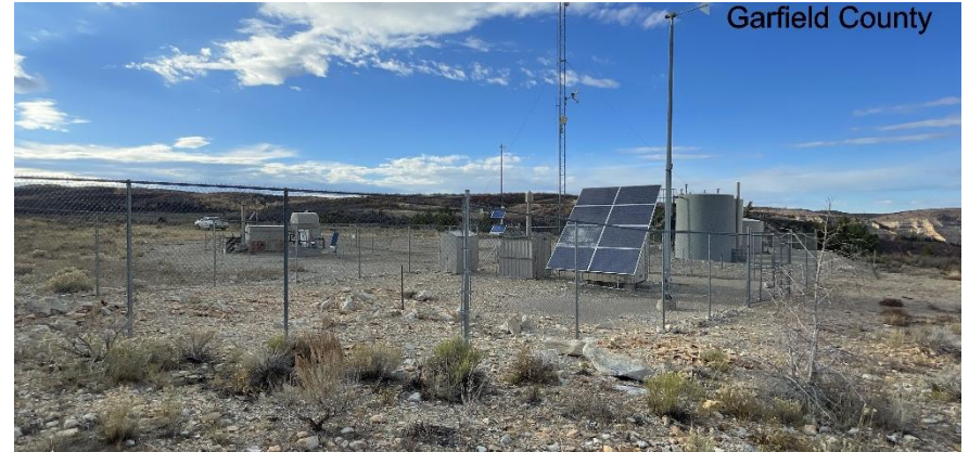
South East corner of location.
