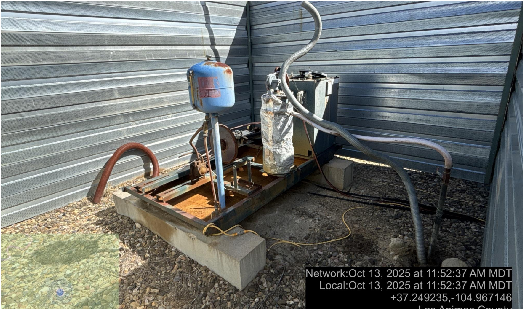
PHOTO 3: UNUSED OR UNUSEFUL EQUIPMENT STORED ON LOCATION (PRIME MOVER SKID HAS NO ENGINE AND IS NOT USEFULL). REMOVE UNUSED EQUIPMENT PER RULE 606. CA DATE 11-13-2025.
