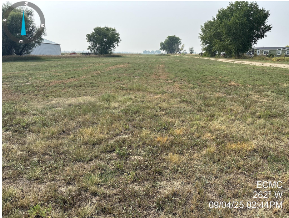
Photo 1. Photo taken of the tank battery location, facing west. Photo illustrates that final reclamation activities have taken place, but vegetation establishment does not appear to meet Rule 1004 standards and weedy annual vegetation including kochia ( Bassia scoparia ) was observed across the location.
