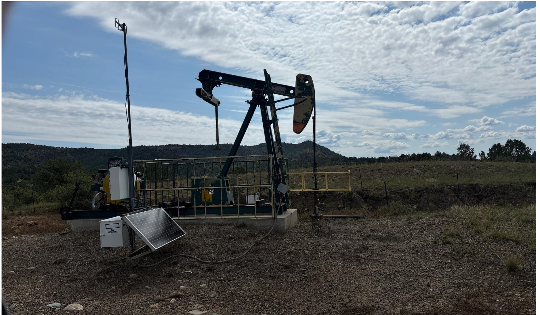
PHOTO 2: WELLHEAD AND EQUIPMENT.
