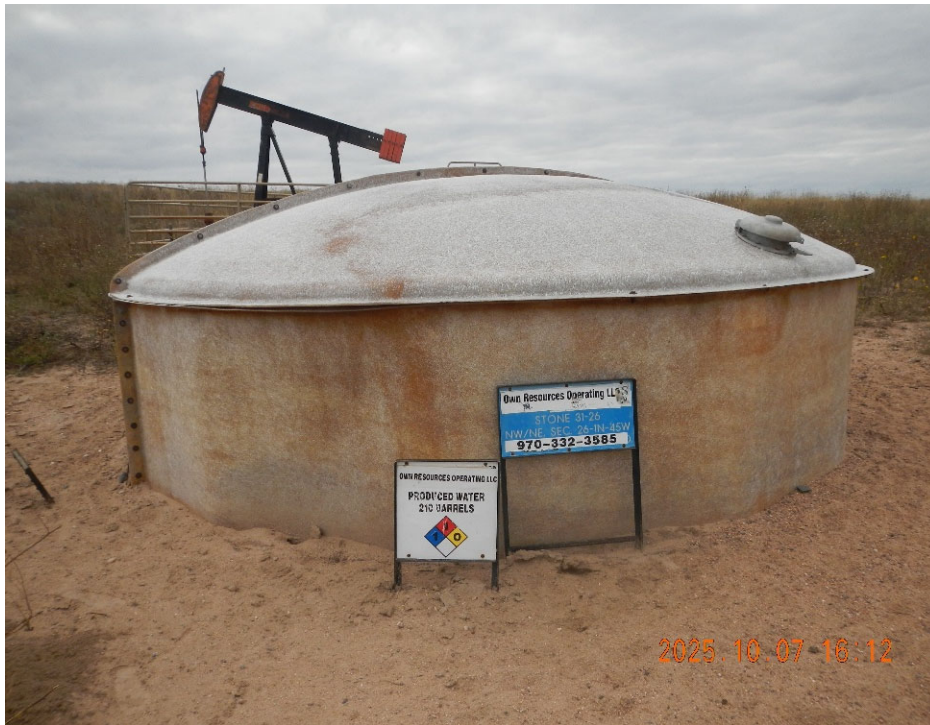
3. View of Production tank at well location.
