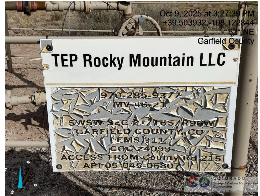
Photo # 5811 Illegible Wellhead Sign
