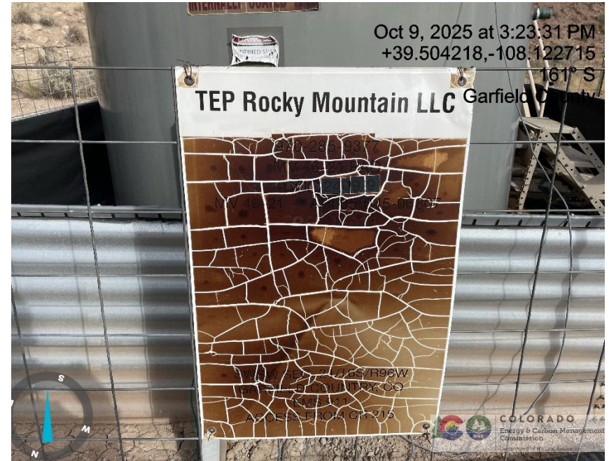
Photo # 5810 Illegible Battery Sign
