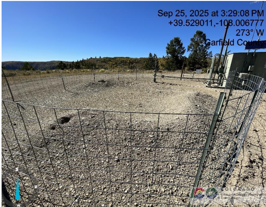
Photo # 3212 From inspection/audit 708907551 conducted on 09/25/2025 Soil stockpile with no BMP's
