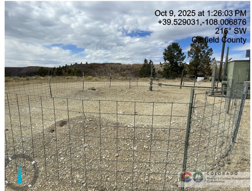
Photo # 5388 Soil stockpile with no BMP's
