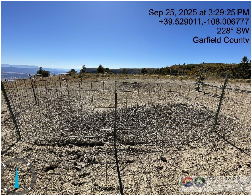
Photo # 3211 From inspection/audit 708907551 conducted on 09/25/2025 Soil stockpile with no BMP's
