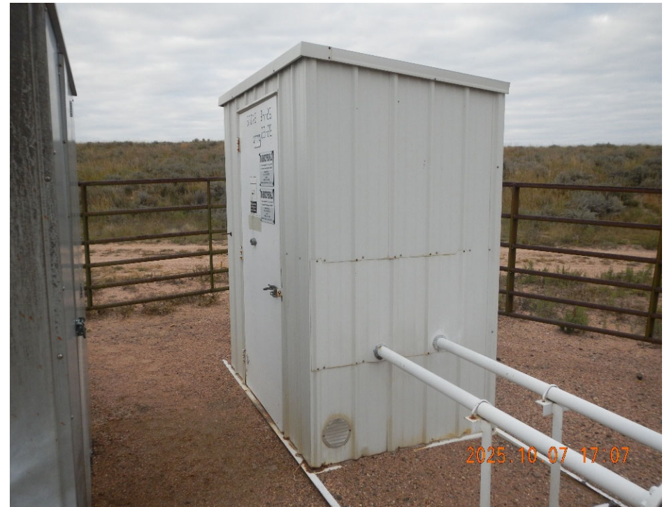
6. View of Gas Meter Run Shed.
