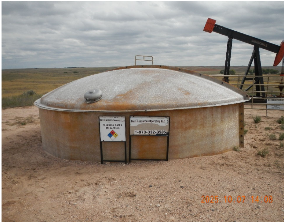
3. View of production tank at well location.
