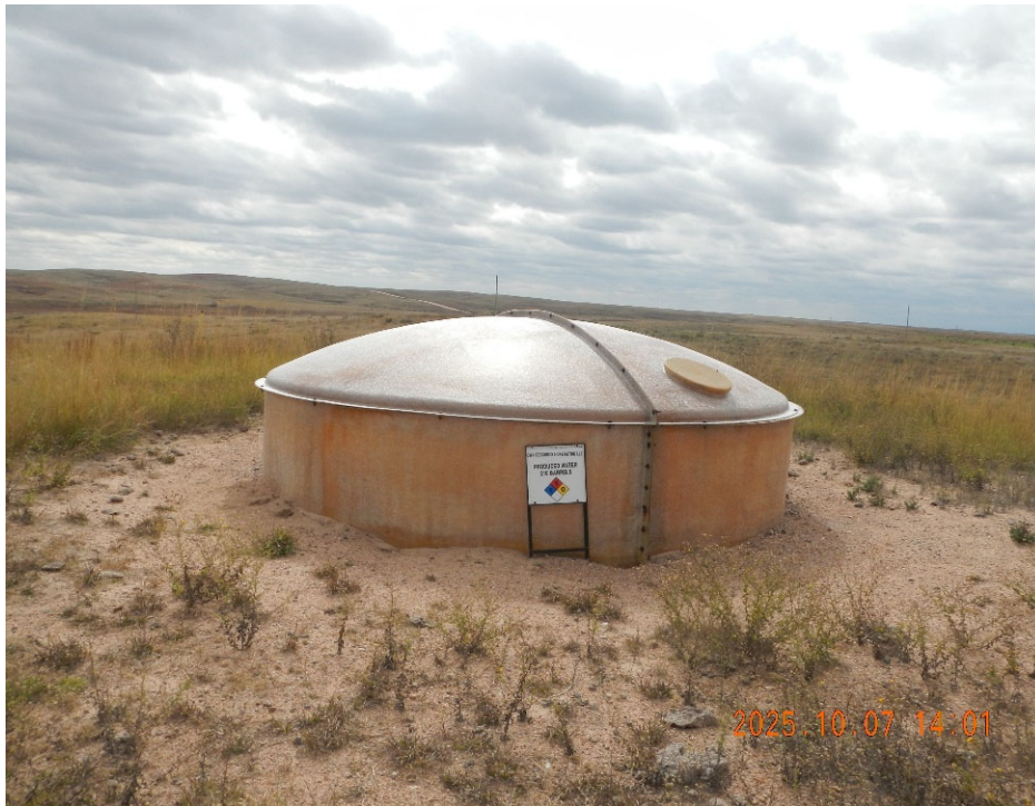
5. View of production tank at well location.
