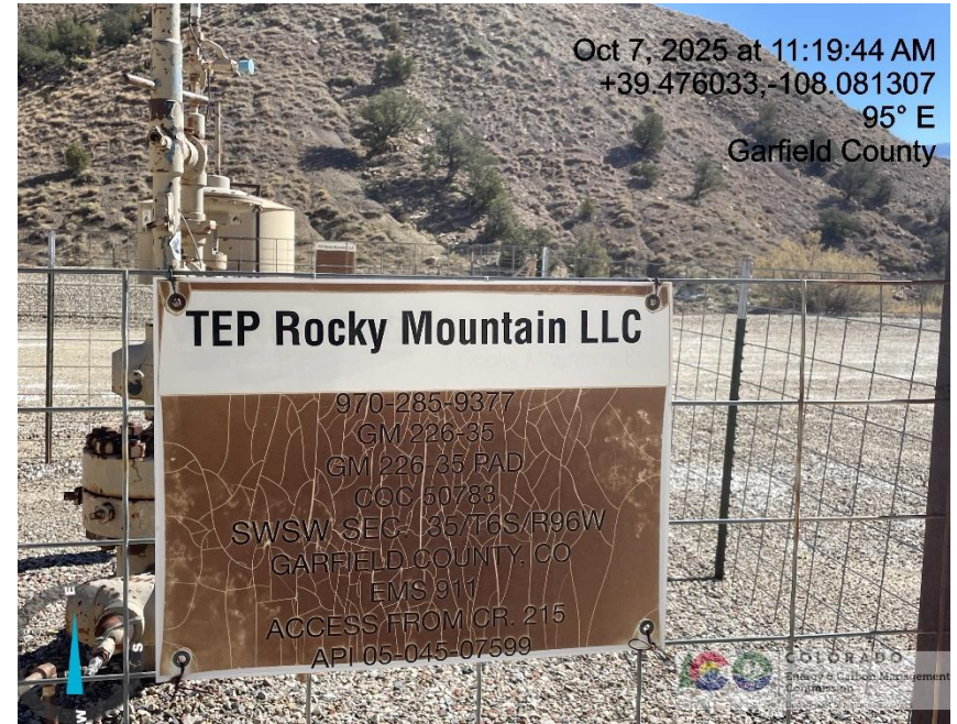
Photo # 4572 Illegible Wellhead Sign
