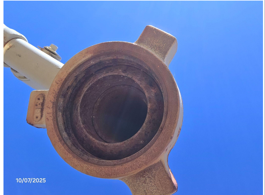
Photo 3: Open ended pipe riser on next to separator equipment.
