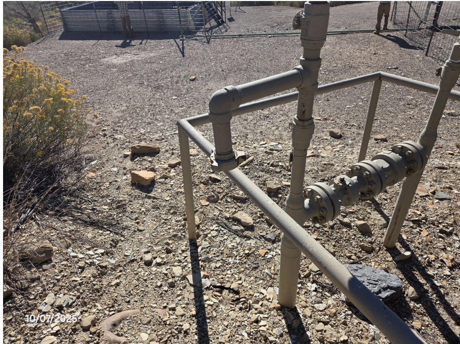
Photo 3: Open ended pipe riser on next to separator equipment.
