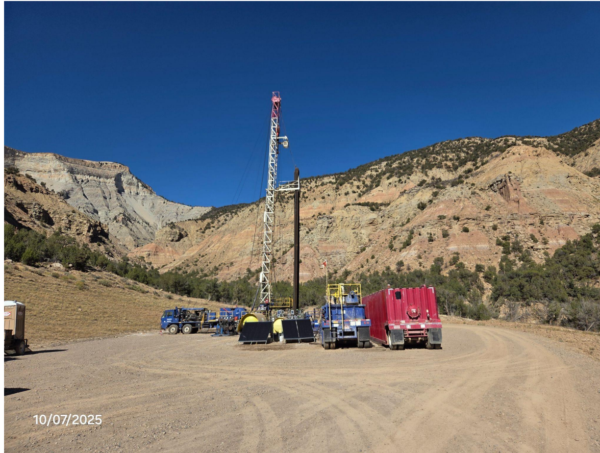
Photo 1: Photo shows work over rig on Location at time of inspection.
