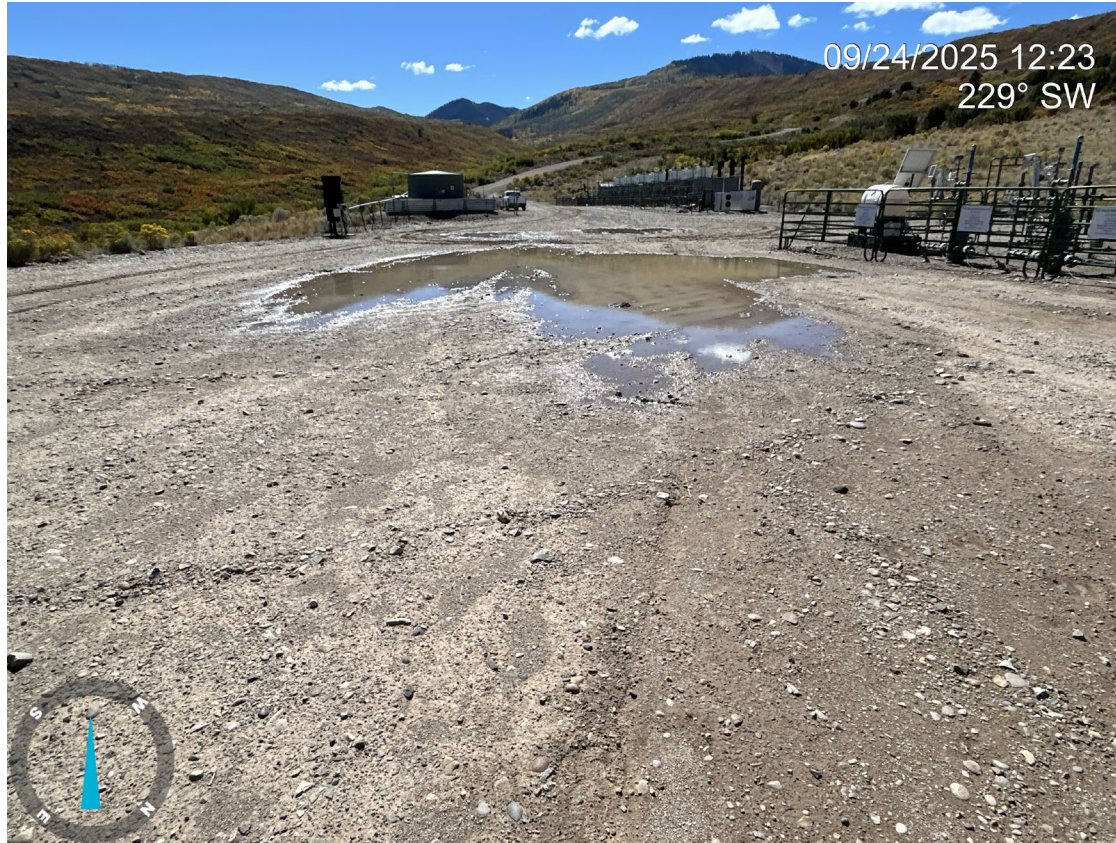
Photo 5: Photo showing ponded water on the working pad surface. Gravel is sparse in some areas. Comply with 1002.f. and implement or maintain stormwater BMPs.
