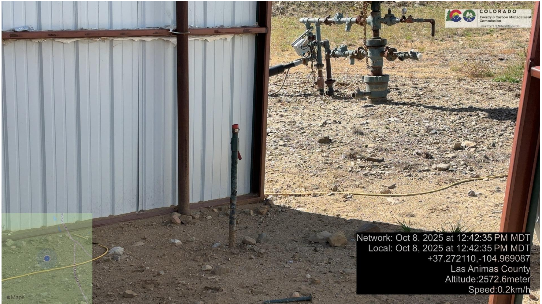
PHOTO 6: UNUSED EQUIPMENT (1" RISER NOT IN USE AND NOT MARKED). REMOVE OR MARK UNUSED EQUIPMENT PER RULE 606. CA DATE 11-8-2025.
