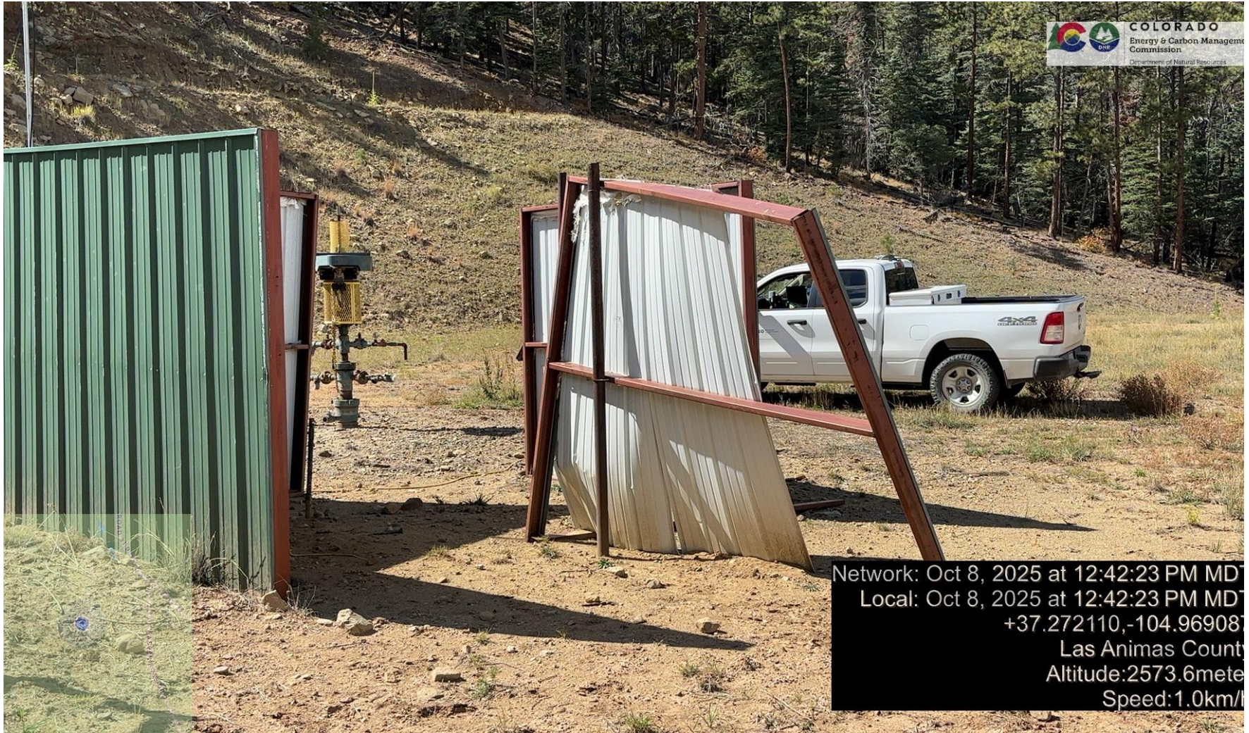
PHOTO 4: UNUSED EQUIPMENT (SOUND WALLS IN DESREPAIR AND NOT IN USE). REPAIR OR REMOVE SOUND WALLS PER RULE 606. CA DATE 11-8-2025.
