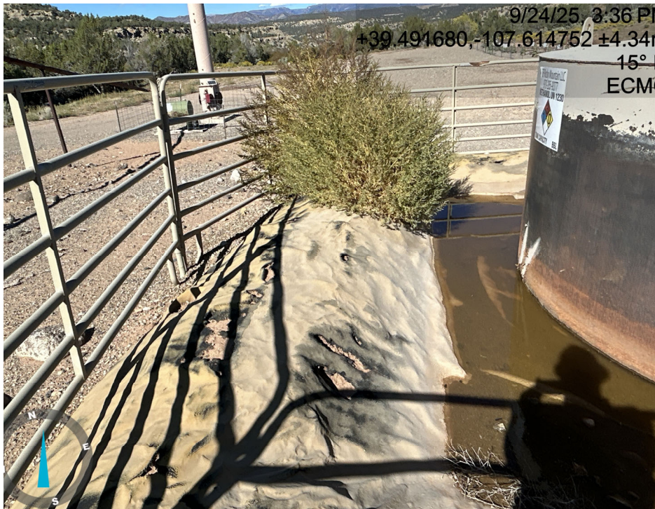
Tank liner has multiple areas with holes, weeds are growing through liner.
