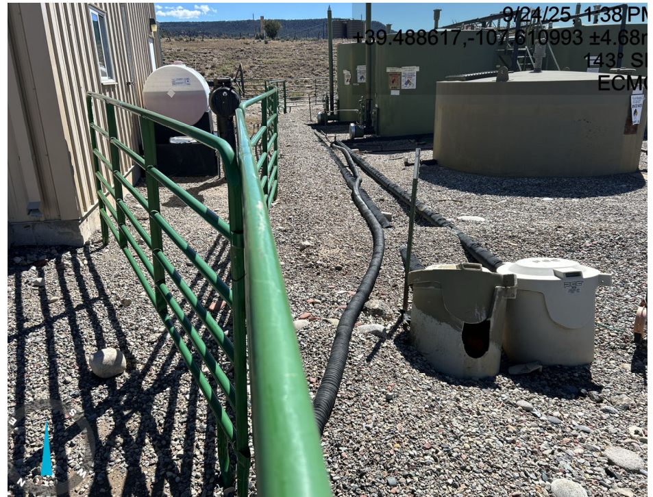
Unused and open-ended hose for wildlife to enter
