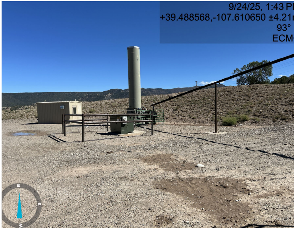
ECD not running and not metered
