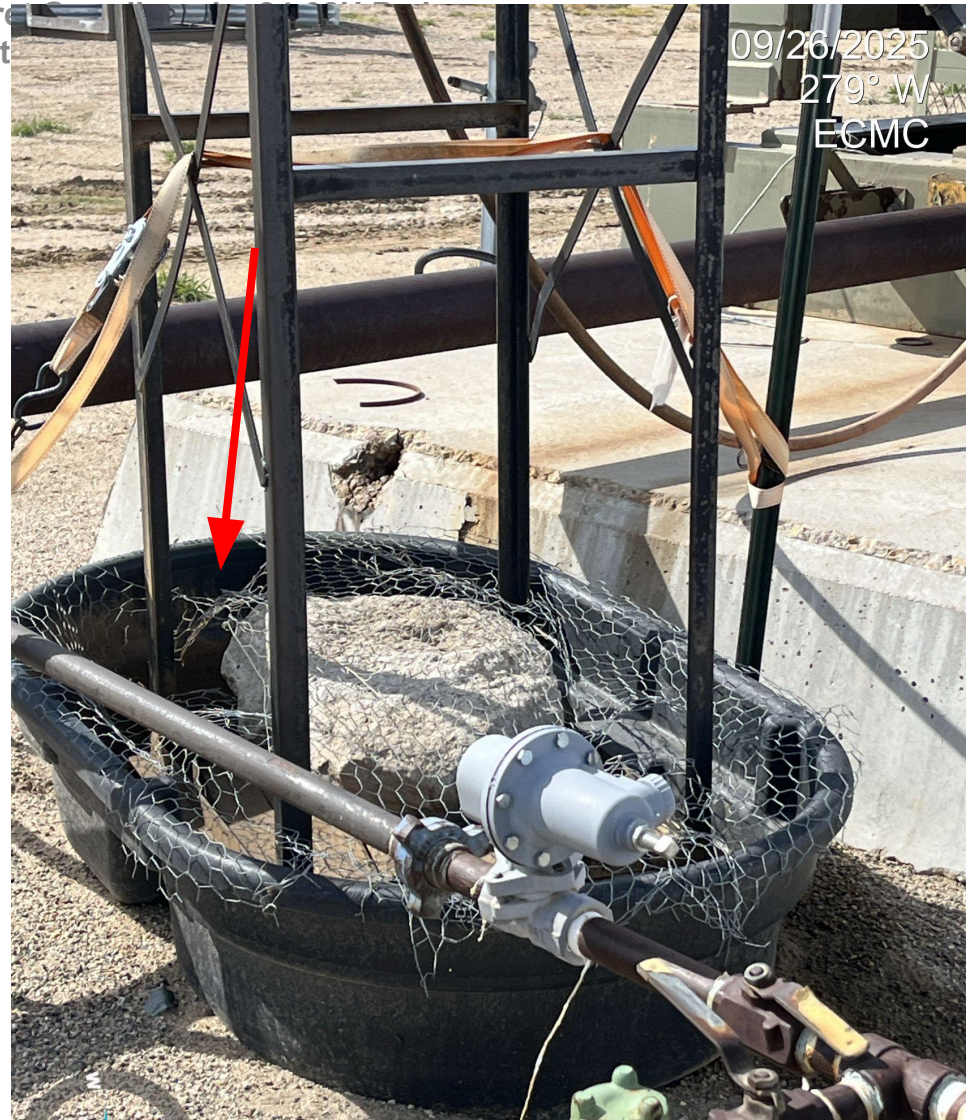
Photo 16. Photo taken of secondary containment at the wellhead, illustrating wildlife protection BMPs are no longer functioning to prevent access to wildlife.
