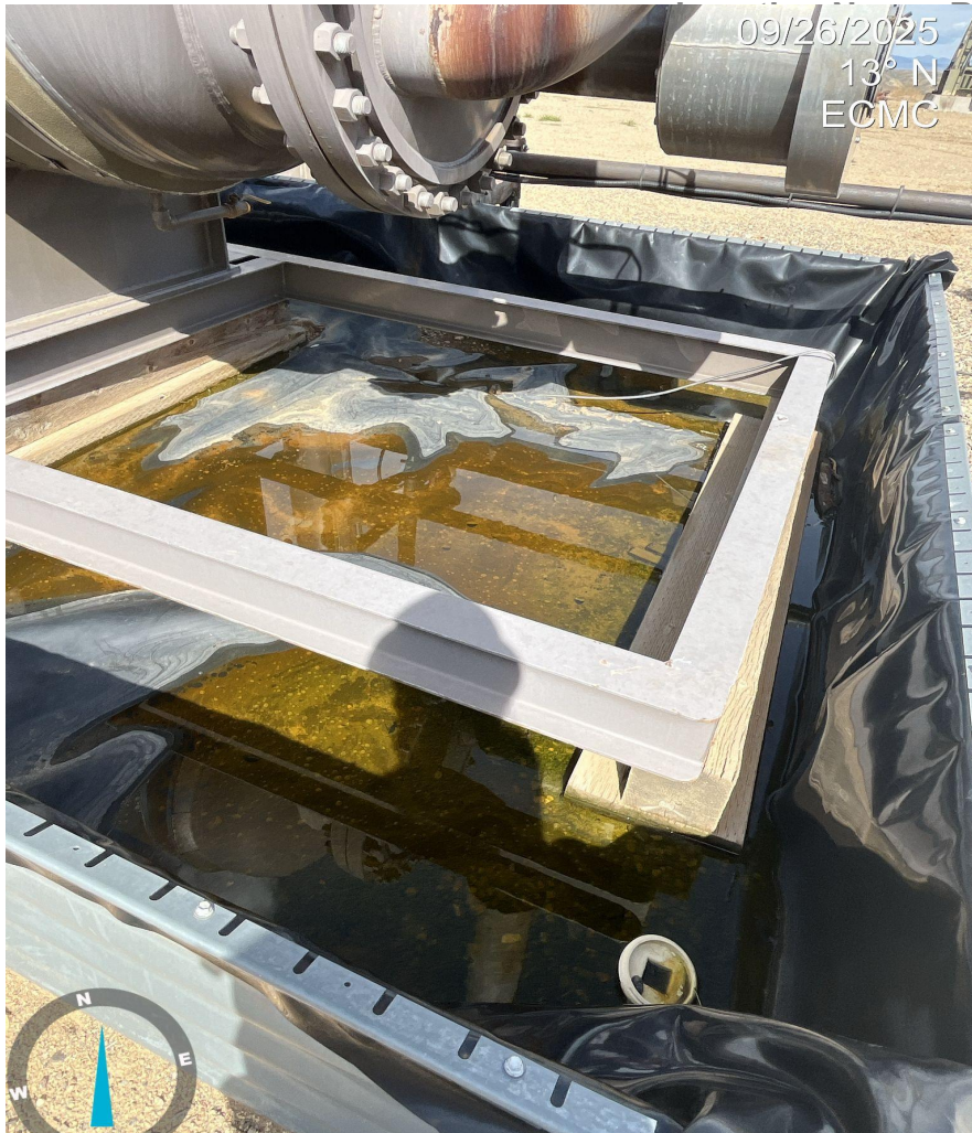
Photo 11. Photo taken at the separator equipment. Photo illustrates fluids inside of secondary containment.
