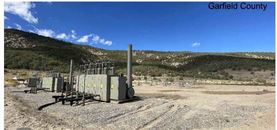
South East corner of location.
