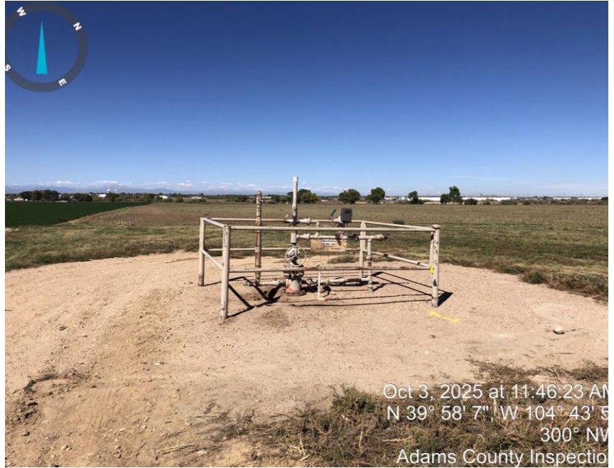
Photo #4 Well head.
