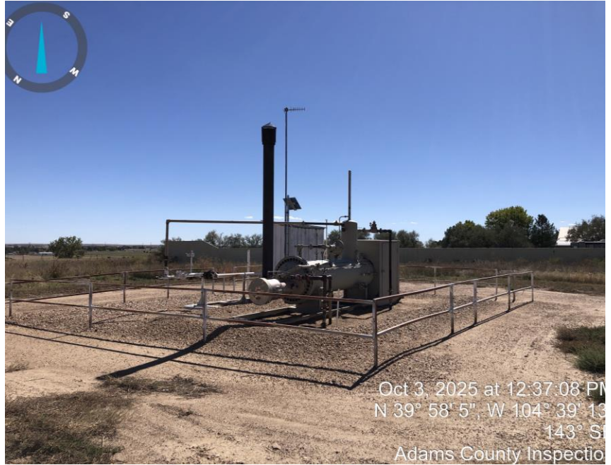
Photo #2 Meter & separator
