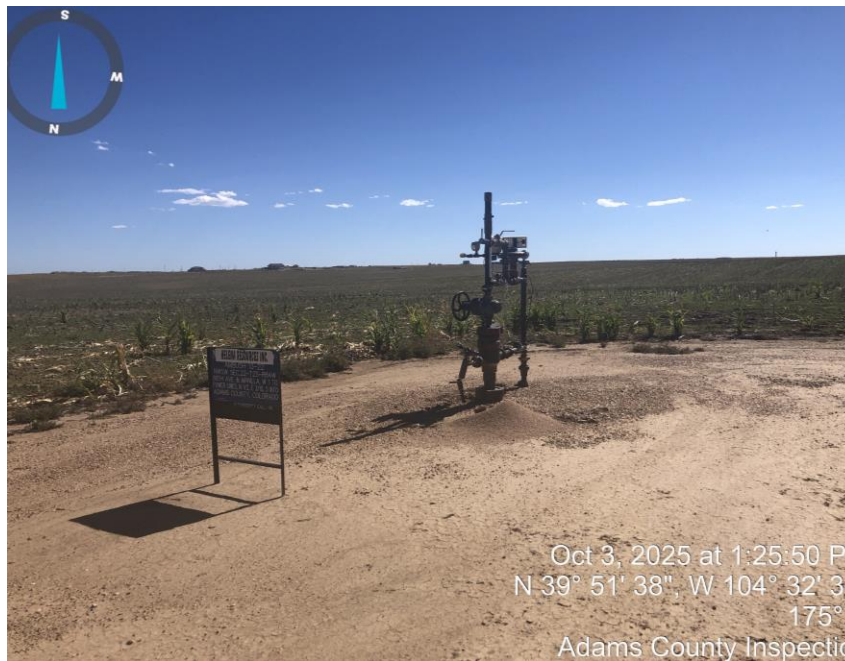
Photo #4 Well head.
