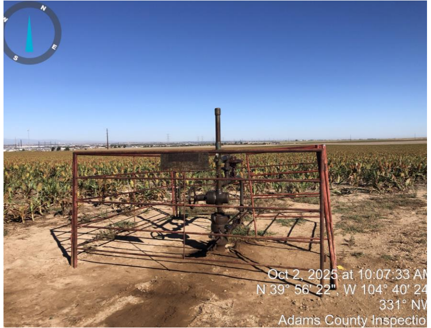
Photo #6 Well head & stained soil.
