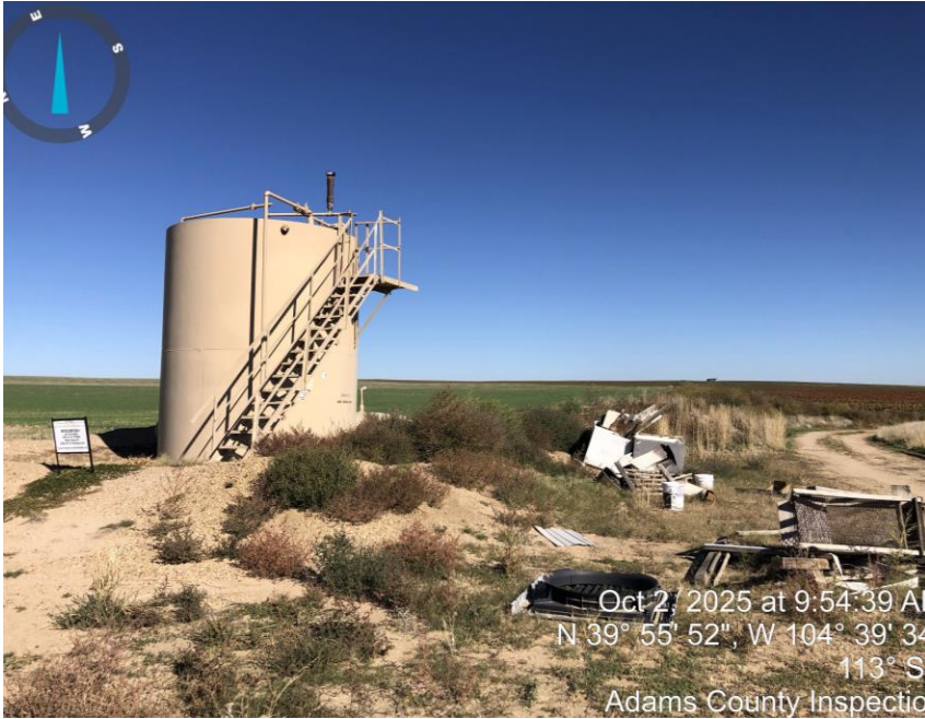
Photo #1 Tanks, weeds & trash.
