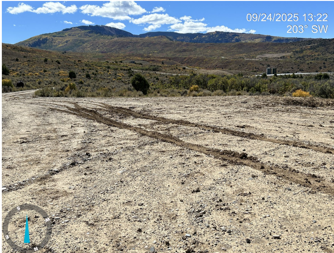
Photo 6: Photo showing an example of vehicle tracking occurring on the working pad surface. Gravel is sparse in some areas on the pad. Maintenance is required. Comply with Rule 1002.f. and implement or maintain stormwater BMP's.
