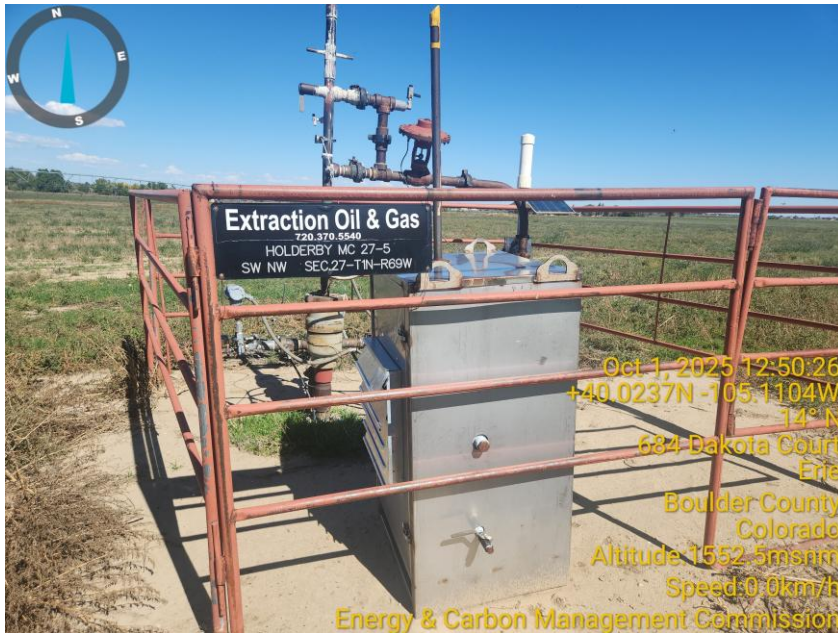
Photo 7 Wellsite sign & Fugitive gas combustion device.
