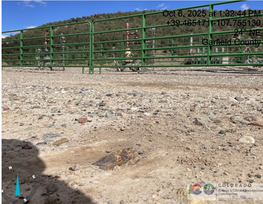
Photo # 4250 Same unmarked deadman
