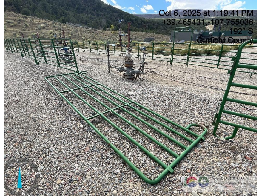
Photo # 4251 Cattle panel laying on ground
