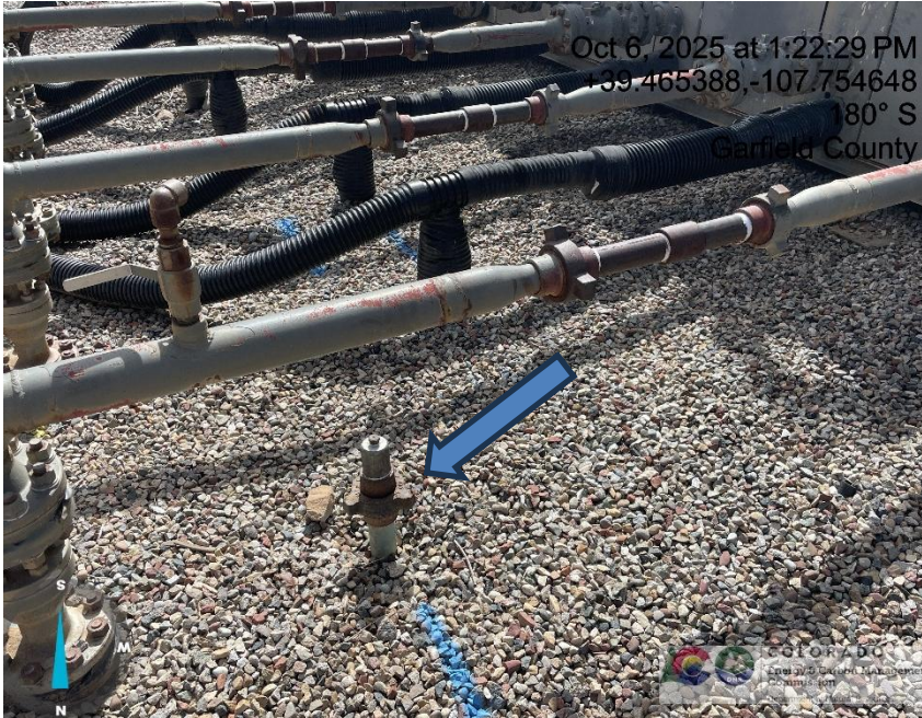
Photo # 4244 Unused flowline lacks lockout tagout (OOSLAT)
