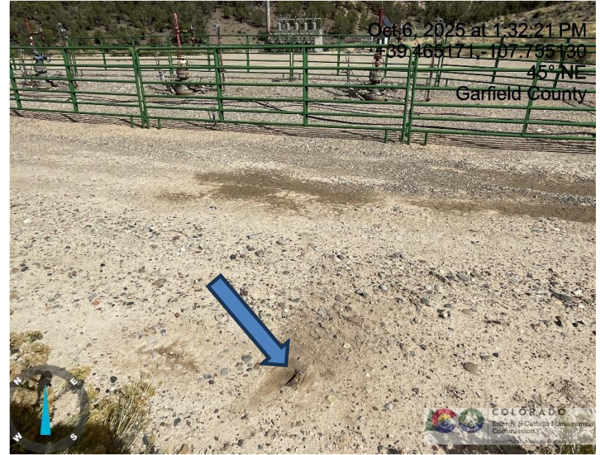
Photo # 4249 Same unmarked deadman
